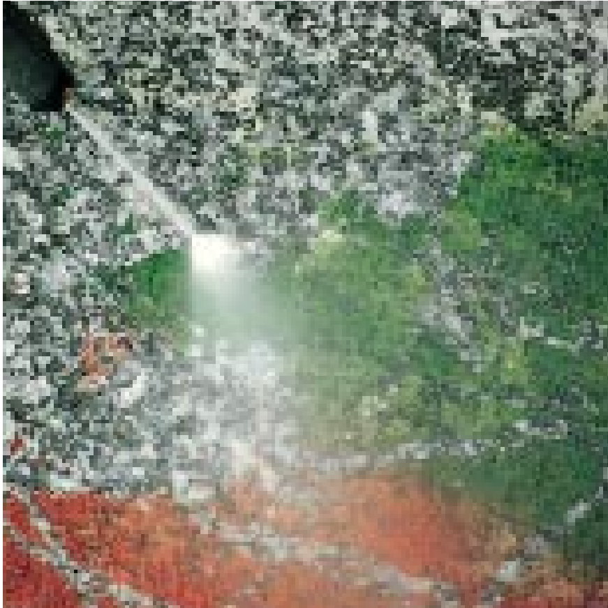
Using a high-pressure cleaner on granite treated with WallGard GRAFFITI BARRIER
