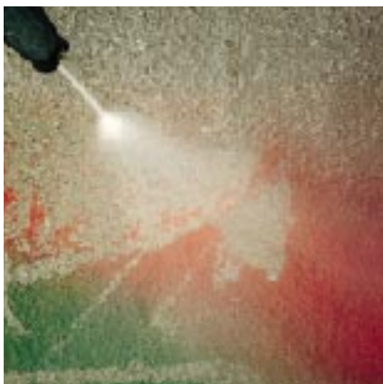
Cleaning concrete treated with WallGard GRAFFITI BARRIER
