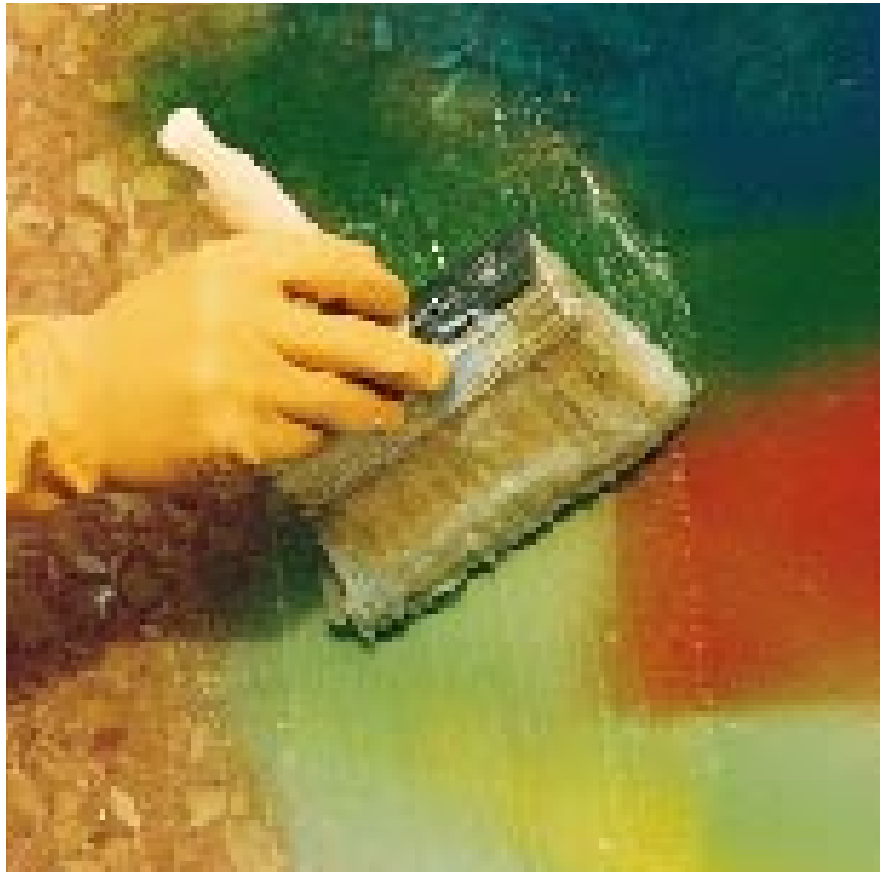
Applying WallGard GRAFFITI REMOVER GEL on natural stone
