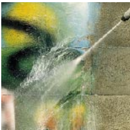
Using a high-pressure cleaner
