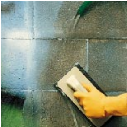
Cleaning with an abrasive pad
