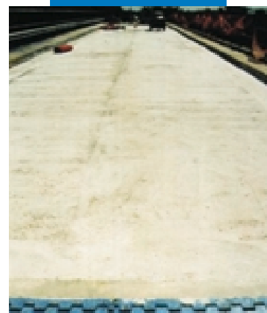
The repaired bridge-deck
