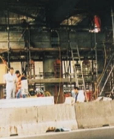
A view of the bridge during repair work
