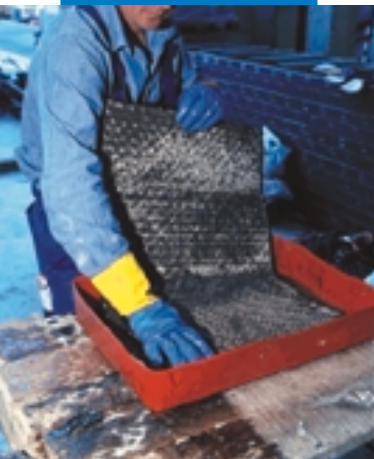
Manual impregnation of Mapewrap C
